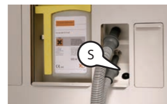
Suction hoses fitted at disinfection nipples.
